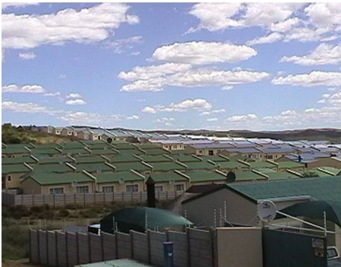
Figure 6 Standardized townhouse complexes have become a dominant feature of suburban developments in Windhoek (photo reproduced courtesy of Brent van Tonder, 2004)
