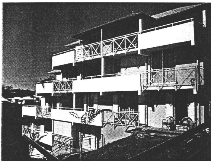
Figure 3 : The "La Découverte" project – northern façade
