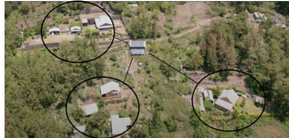
Fig. 1. Drone photography of the case study microgrid.
