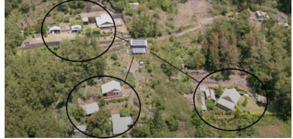
Fig. 1. Drone photography of the case study microgrid.
