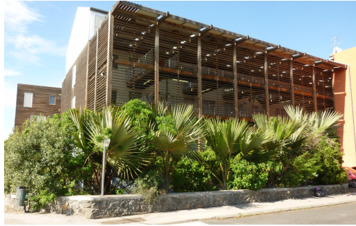
FIGURE 1. Overview of the North facade of the case study : green patio with large solar protections
