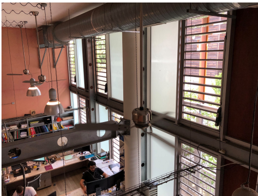
FIGURE 2. View of the louvers and ceiling fans in open-spaces
