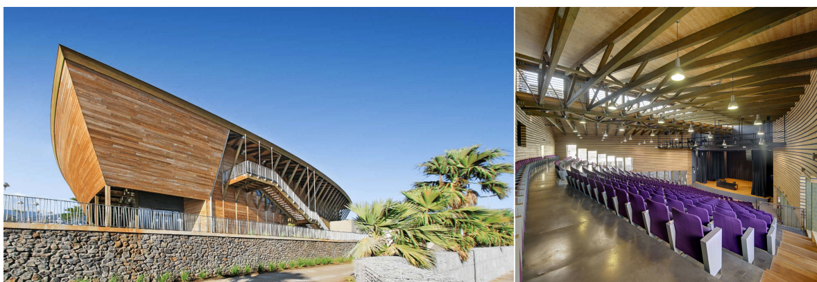
Figure 7: First natural ventilation based bioclimatic amphitheater under tropical climate.
