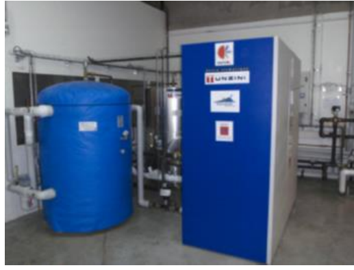
Fig. 1. RAFSOL installation with, on the roof, the solar collector field and the cooling tower (left) and, in the technical room, the absorption chiller and the 2 buffer tanks (right).
