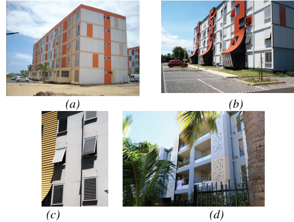
Figure 3: Retrofitting of an existing large tower block ‘Bons Enfants Building C’ and passive solutions set up: (a) South façade of the old existing building, (b) same façade for the retrofitted one, (c) louvered shutters and (d) exterior covered veranda. Photo Credits: T. Giraud.
