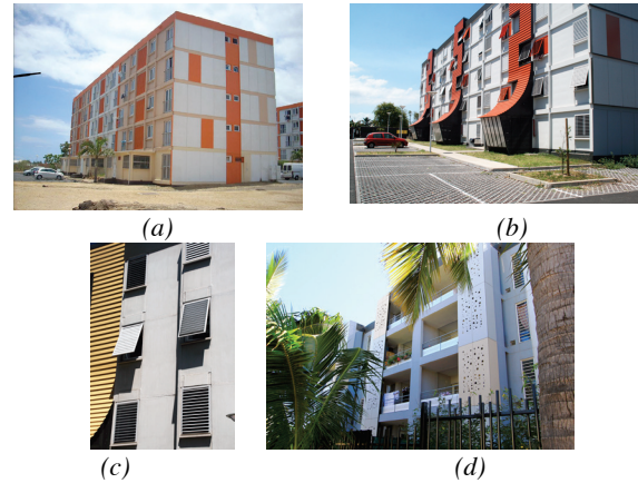
Figure 3: Retrofitting of an existing large tower block ‘Bons Enfants Building C’ and passive solutions set up: (a) South façade of the old existing building, (b) same façade for the retrofitted one, (c) louvered shutters and (d) exterior covered veranda. Photo Credits: T. Giraud.
