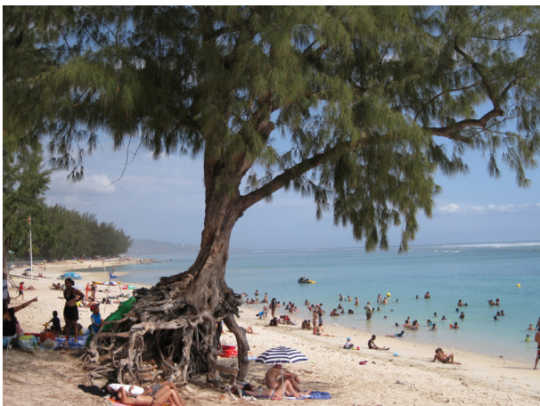
Fig. 9. Root-exposed filao trees on L'Ermitage beach, in danger of toppling
